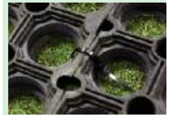
Connect matting together with cable ties.
