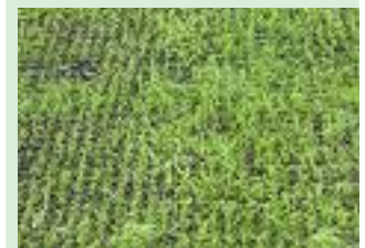
Allow the grass to grow through the mesh apertures.
