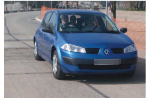
BodPave ® 40 used as the vehicle access roads
