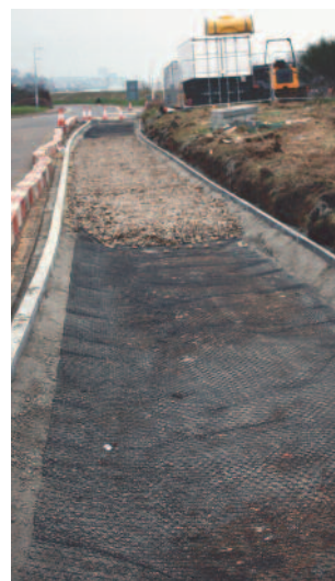
Installation of BodPave ® 85
