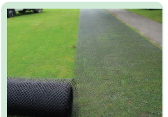
Mesh laid onto existing grassed surface
