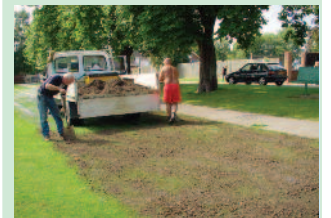
Topsoil brushed over the surface
